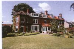
Fig. 6: Middlecave Lodge (south facing elevation).
