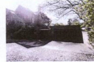
Fig. 11: Existing garage block (north facing elevation) and Middlecave Lodge (left of frame).
