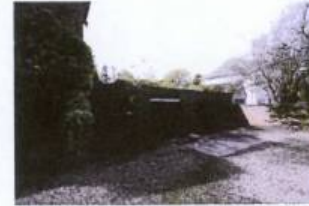
Fig. 10: Existing garage block (north facing elevation) and adjacent steps to Middlecave Lodge, with No. 75 beyond.
